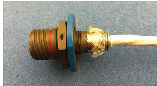
Figure 43: Placing the washers near the connector
