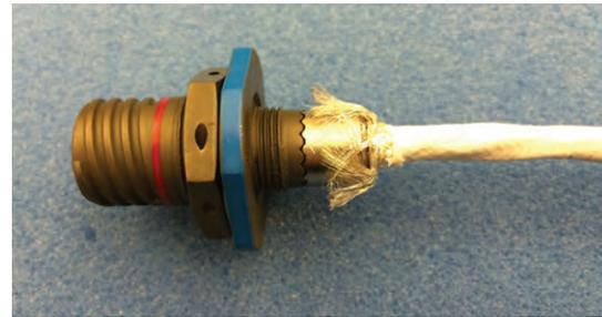
Figure 42: Trimming the excess braid material
