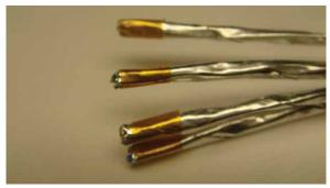
Figure 47: Taping each pair
