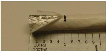
Figure 44: Slitting the cable jacket
