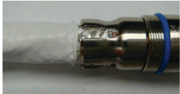
Figure 23: Trimming the outer jacket
