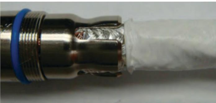
Figure 40: Trimming the outer jacket
